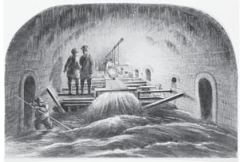
The Fleet sewer.
